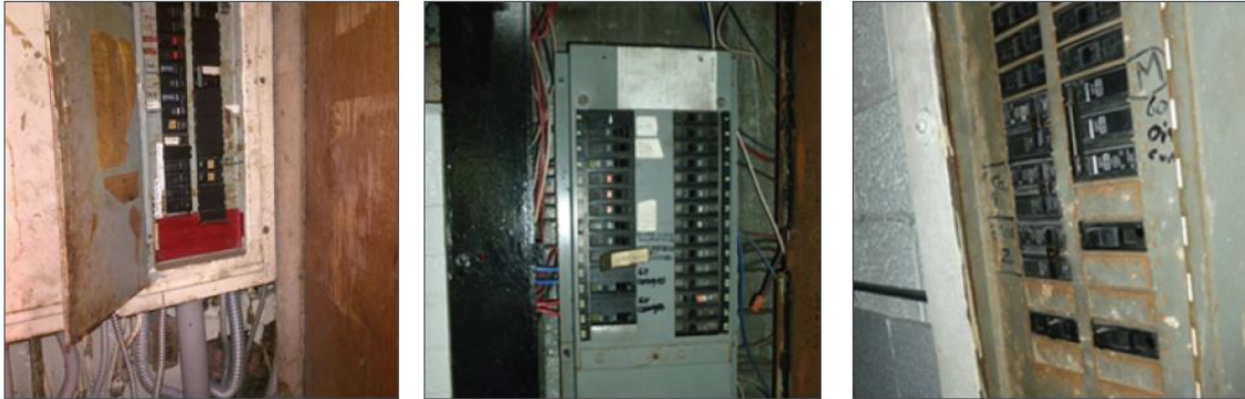
Figure 10 Older electrical panels, such as these examples, may require upgrades to meet today's electrical codes Courtesy Energetics Incorporated
